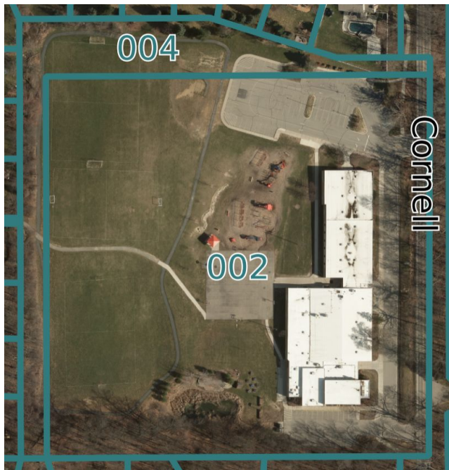
Cornell Elementary Site
